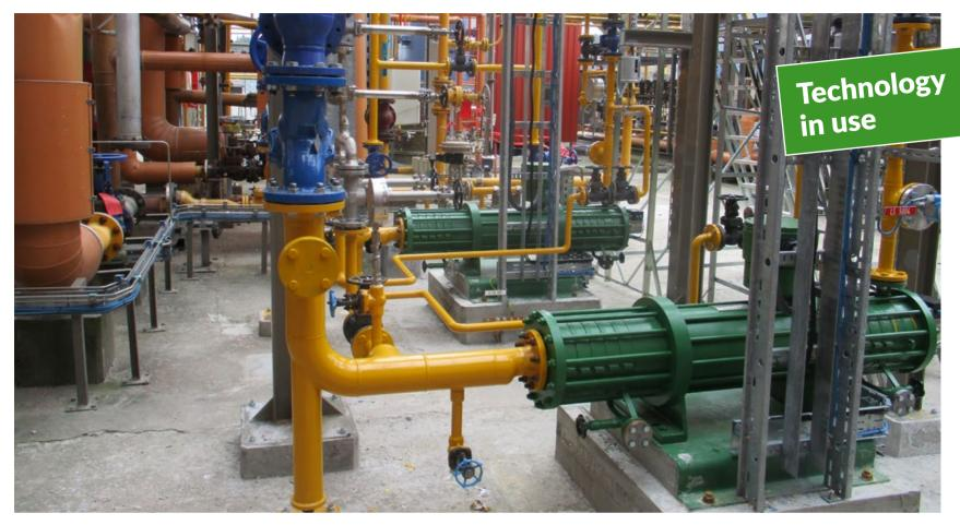
Canned motor pumps with tandem design
